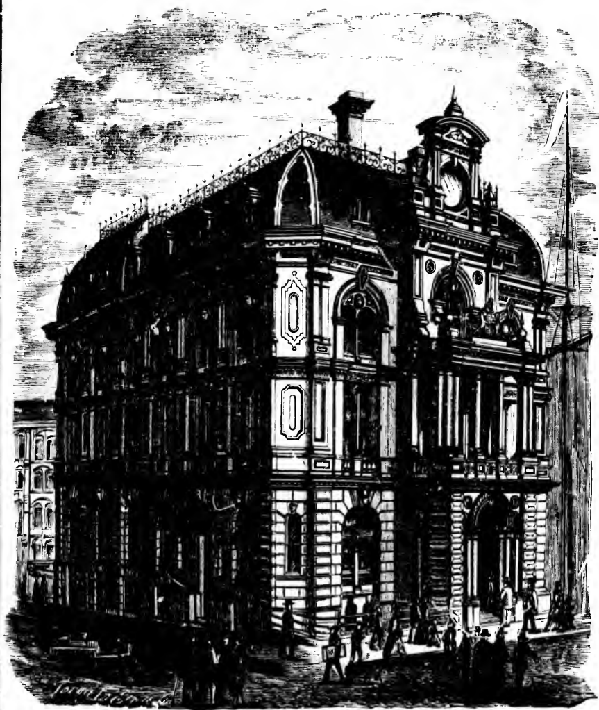
CUSTOM HOUSE, TORONTO.
